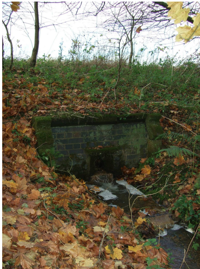
Photograph 23 Old outfall to stream at eastern end of valley feature
