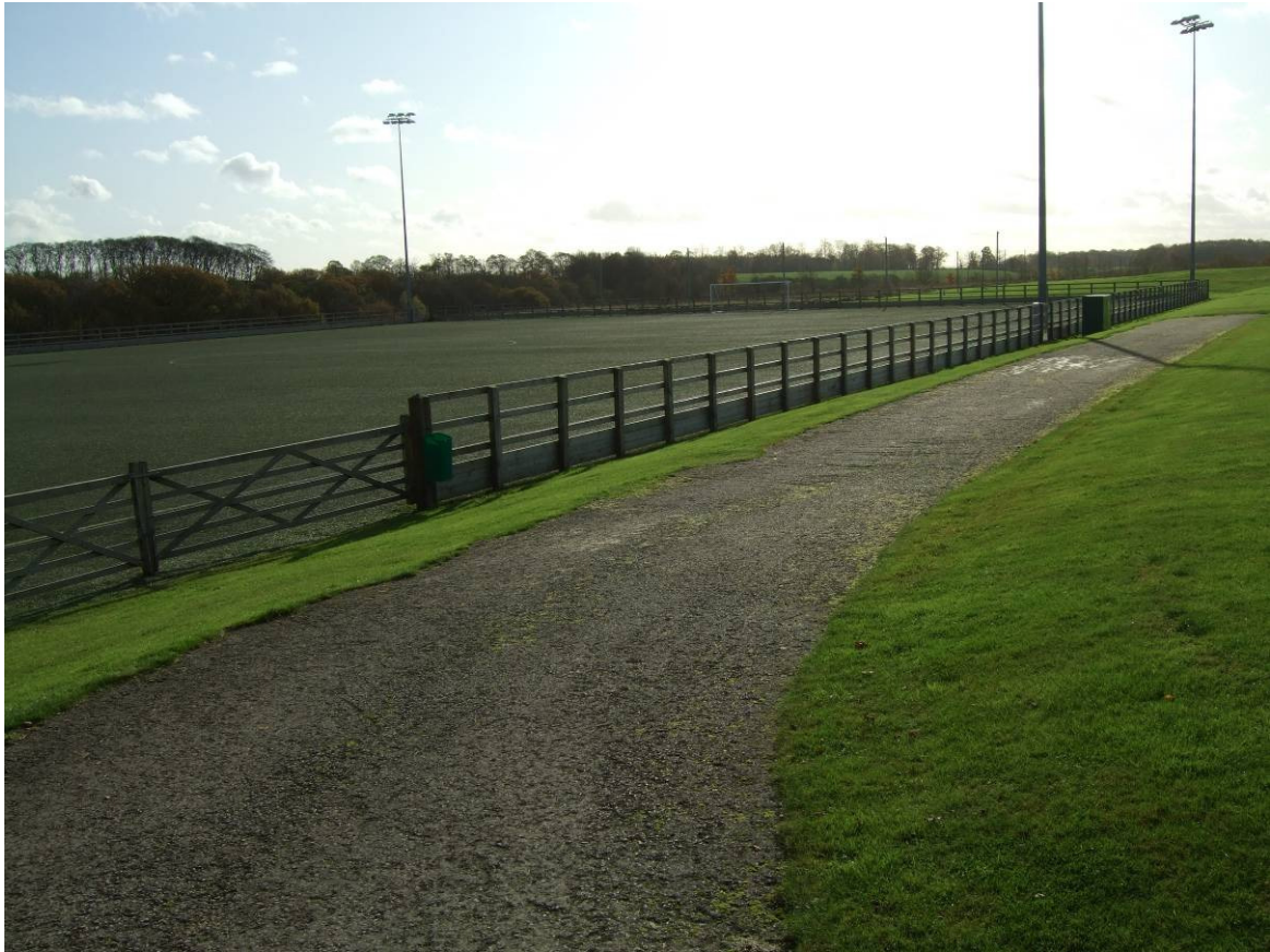
Photograph 24 Panorama across south eastern corner of site showing area around existing artificial pitch
