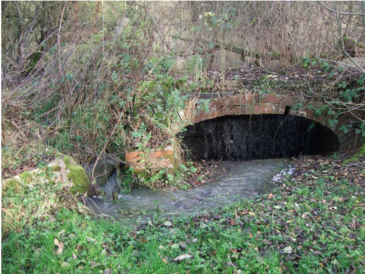
Photograph 22 Brick weir below southern pond showing water flowing around weir
